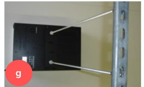
Any fine adjustments can be made at this stage as the nuts and the threaded bar will take the weight of the Smoke Screen.
