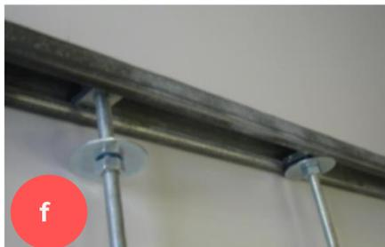
Fix the unistrut into place. There are a range of fixings to accommodate concrete ceiling, girders etc.; if in doubt contact the fixing supplier. Attach the threaded bar to the unistrut using the channel nuts, 38mm washers and M8 nuts. Once this is done the Smoke Screen can be lifted into position and the set screws tightened as above.
